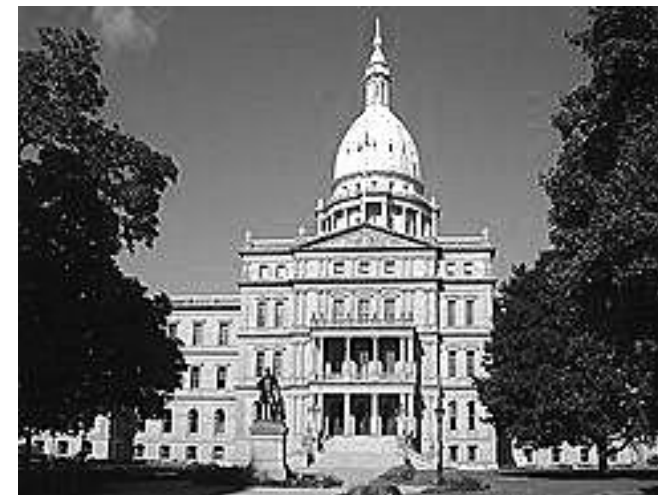
STATE OF MICHIGAN CAPITOL BUILDING PHOTOGRAPHER: BRIAN CHARLES WATSON
